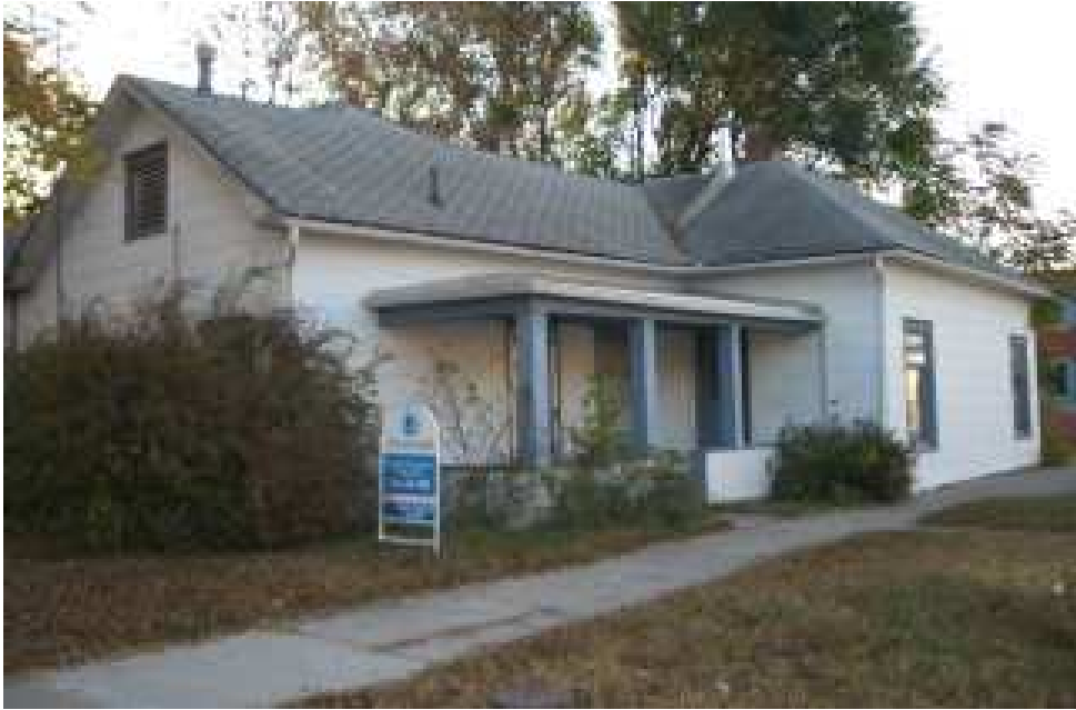
General Repair Needed
